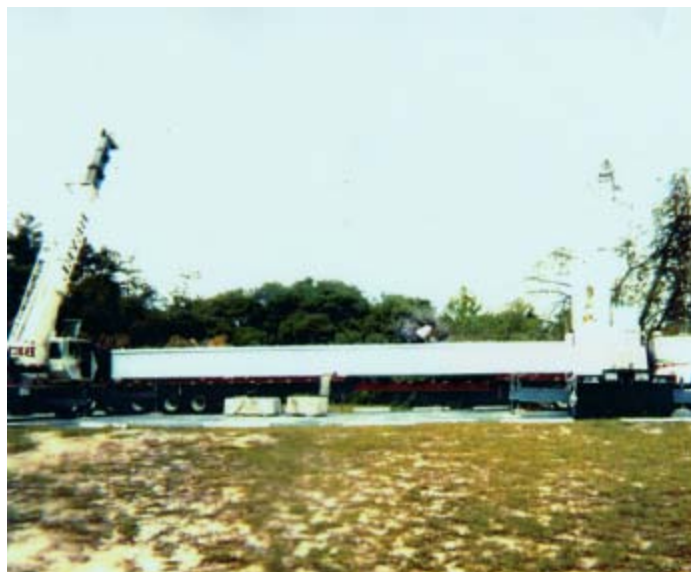
Figure 19. Photo of 72 Foot Long Monorail Guideway Beam Delivered to Maglev-2000 Facility in Florida From Construction Site in New Jersey
