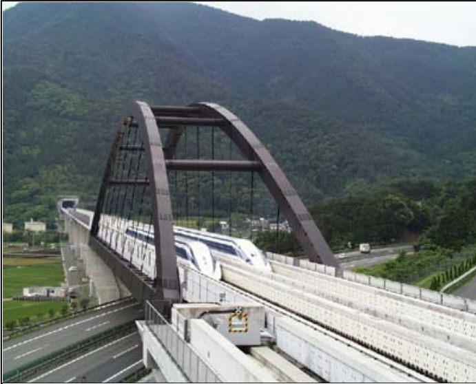
Figure 1 View of Japn Railways Superconducting Maglev Guideway and Vehicle System
