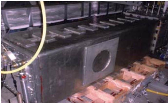
Figure 12. Completed Maglev-2000 Quadrupole Enclosed in its Cryostat
